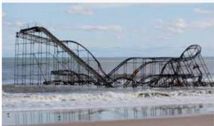
Hurricane Sandy ... npr.org
